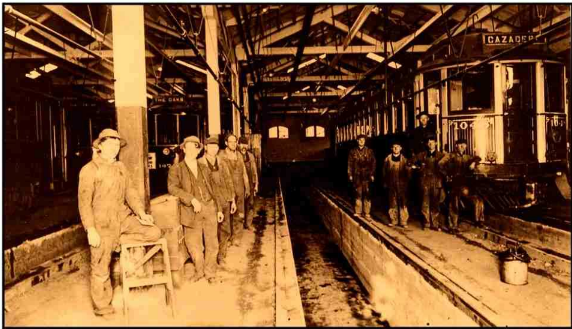
Interior view showing the crew at the Sellwood Car House.
