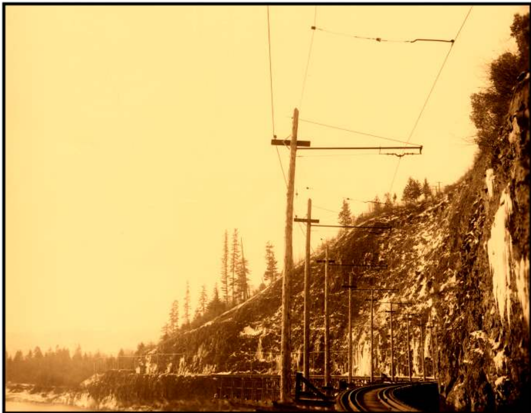
Falling rocks frequently obstructed the tracks and occasionally damaged the trains on the 1400-foot Elk Rock Trestle which opened in 1888.
