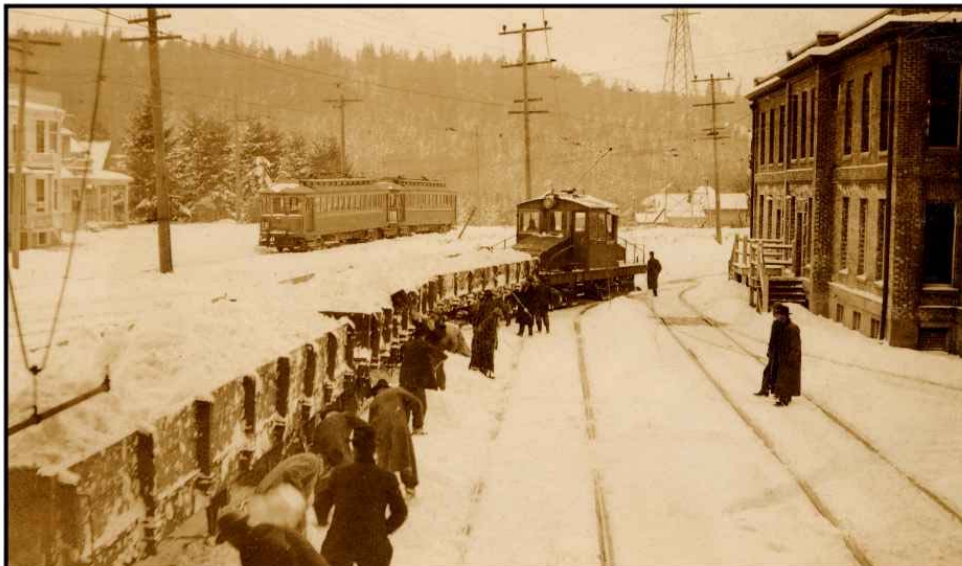
Early winter view of the Motormen's Club House (right) at the Sellwood Car barn.
