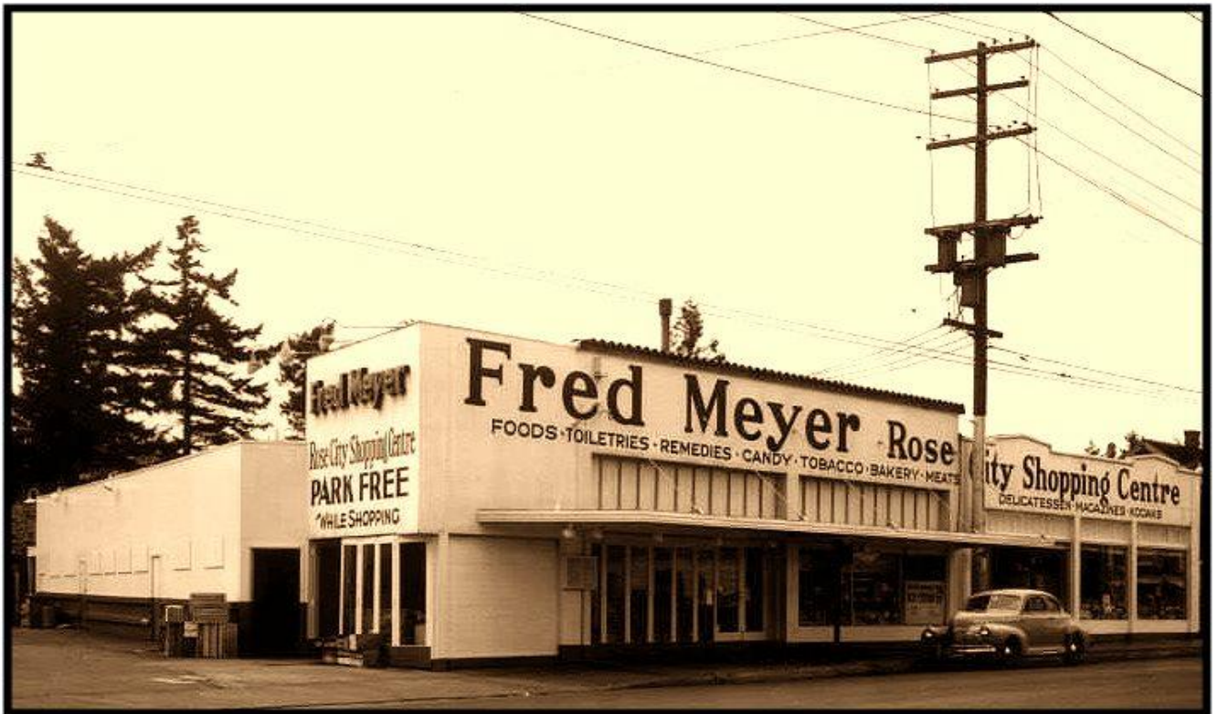
The Fred Meyer Rose City Shopping Centre at 72nd and NE Sandy Boulevard opened in the 1940's.
